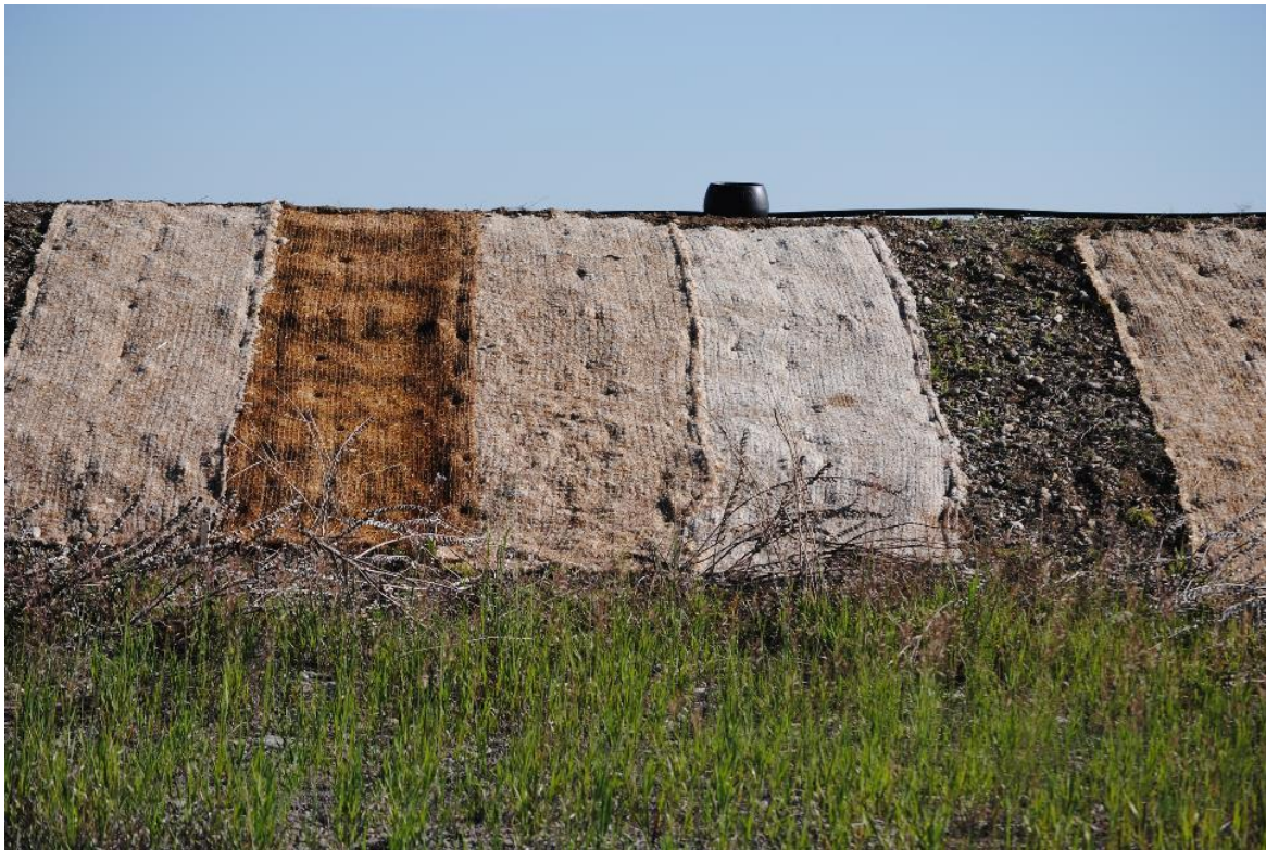
Figure 18: One replication of the six treatments at the Transcend test slope.
