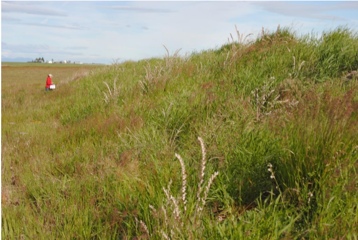
Figure 20: Overview of the Transcend test slope vegetative cover, June 2017.
