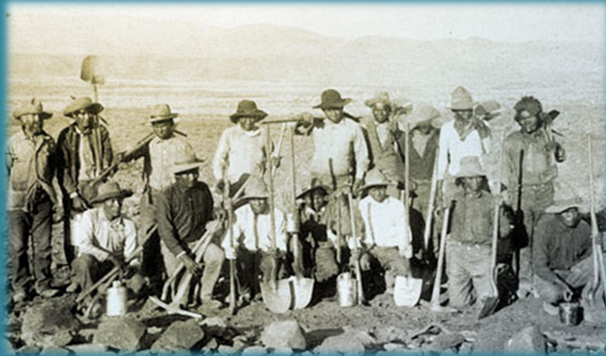
Roosevelt Dam Road Construction Crew 1906
