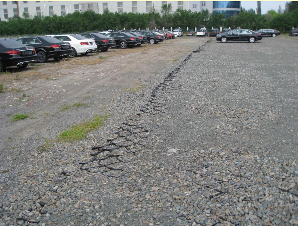
Gravel parking lot
